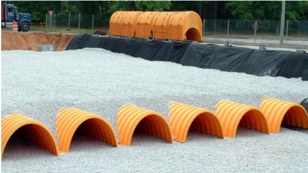
Fig.23 - Voided Arch Attenuation System
